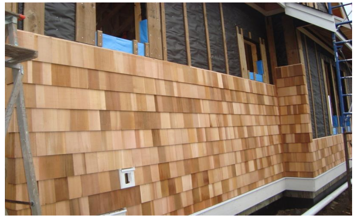
Above is typical installation to rainscreen strapping
